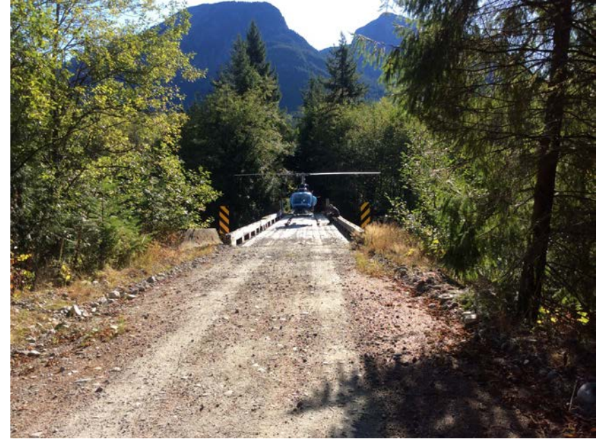
Approach from Right Bank when facing downstream
