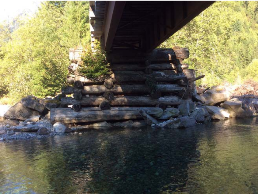
Right Bank Abutment when facing downstream
