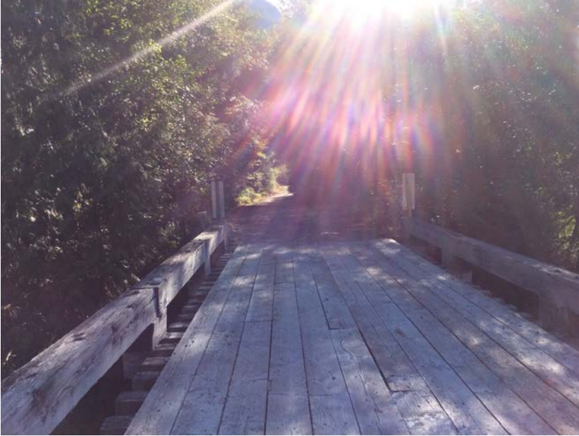
Left approach viewed from bridge
