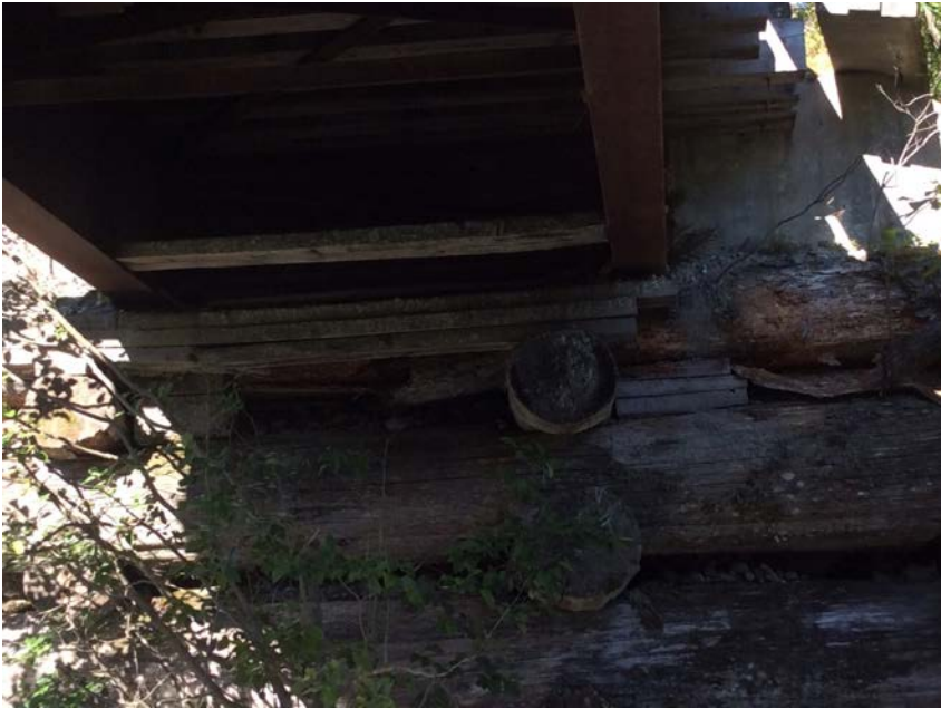
Right Bank Abutment when facing downstream
