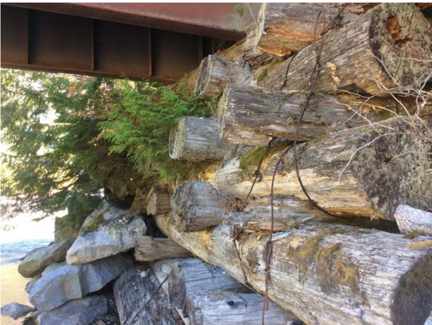
Left Bank Abutment when facing downstream
