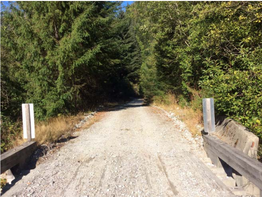
Right approach viewed from bridge
